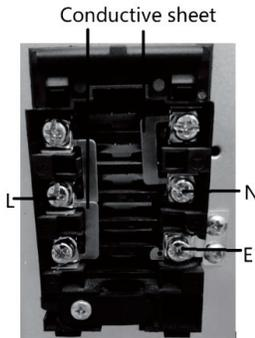
2, 380V-415V 2N~: power cord requirements: wire diameter 4G 4.0mm<sup>2</sup> at least; cord type:
